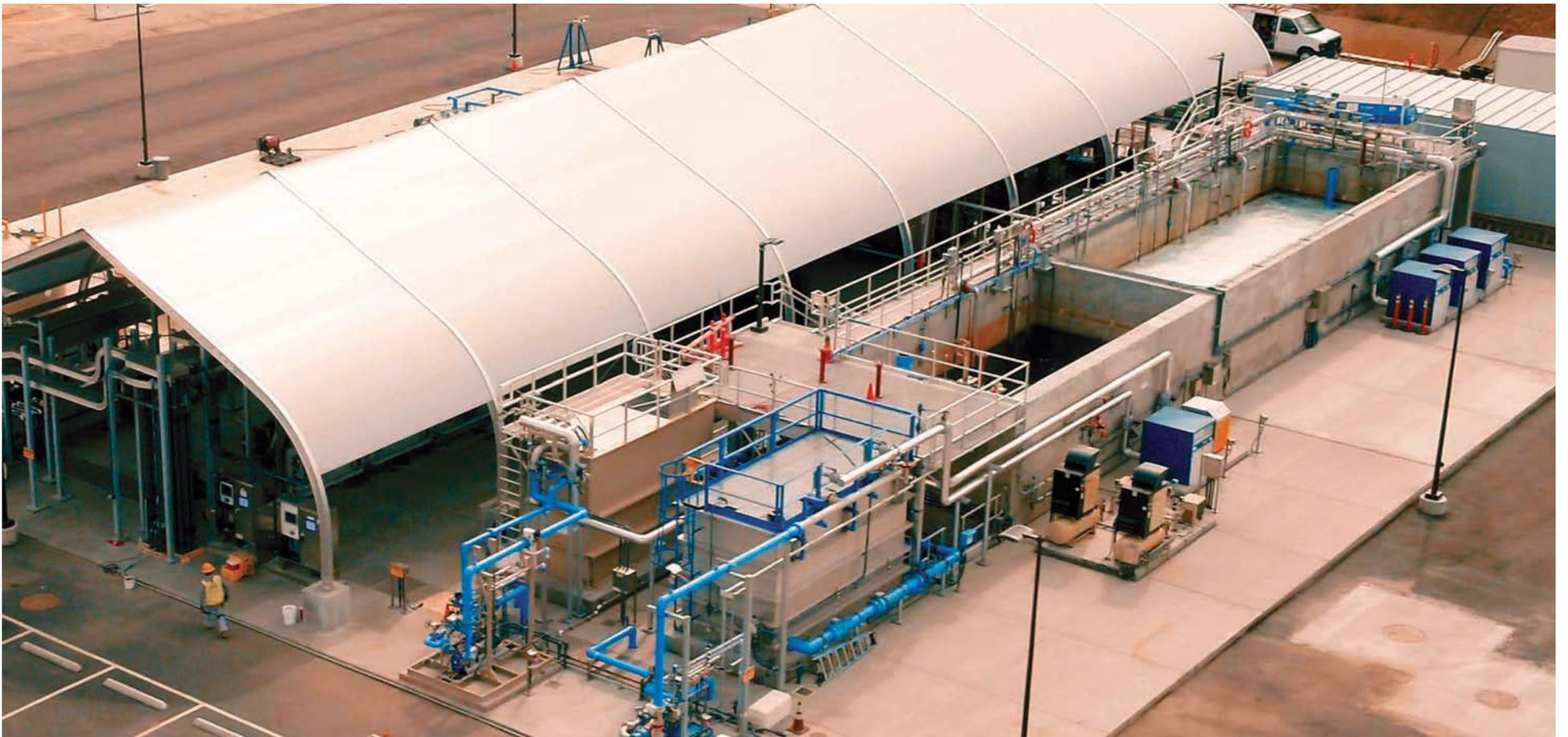
Located in Carson, this demonstration facility purifies 500,000 gallons of treated wastewater per day by using membrane bioreactors, reverse osmosis and ultraviolet light to remove bacteria, minerals and other chemicals. A full-scale facility would make the region less dependent on imported water. *Photos courtesy of the Metropolitan Water District of Southern California*
